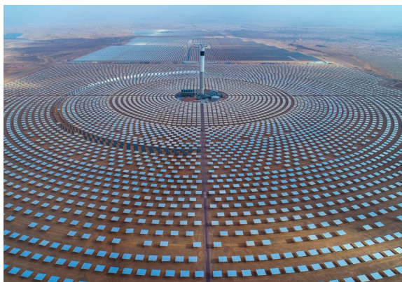
Part of Morocco's NOOR II and NOOR III Concentrated Solar Power (CSP) project in Ouarzazate, Morocco. Photo credit: Xinhua / Alamy Stock Photo.
